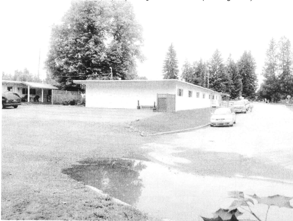
View of north side of subject property along vacated ROW (Looking West)
