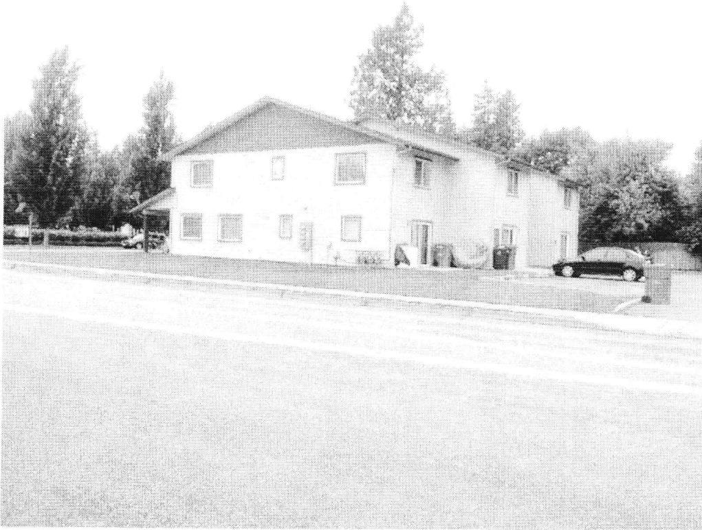
4-plex along 23 rd St. (looking SW from Port of Hope)
