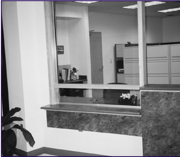
Receptionist's window with a sliding opening to receive items from the public. (Photograph courtesy of Voorhis Robertson Justice Services.)
