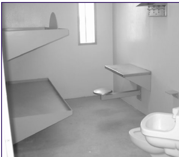
Double-occupancy cell in a direct supervision facility with fixed desk and porcelain fixtures.
