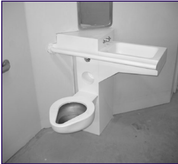
Specially designed toilet and sink combination unit with grab bars for use by inmates with disabilities. (Photograph courtesy of Liebert & Associates.)
