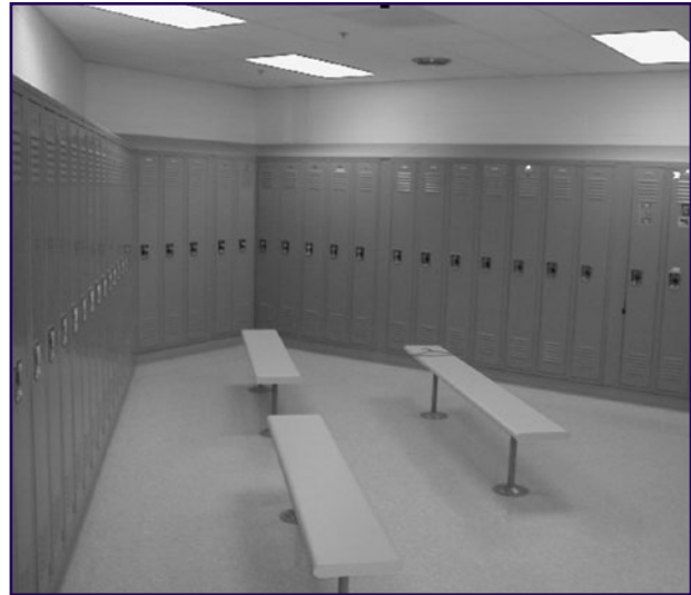
Locker room in a smaller jail. (Photograph courtesy of Liebert & Associates.)
