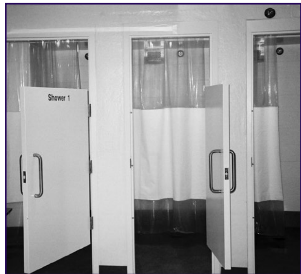
Showers in a housing area with both a door to the dressing area open at the top and bottom and a shower curtain that is clear at the top and bottom for the shower area.
