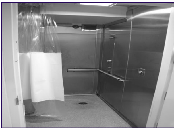
ADA-compliant shower with grab bars, a retractable seat (located behind the curtain), and dual-height shower heads. (Photograph courtesy of Voorhis Robertson Justice Services.)
