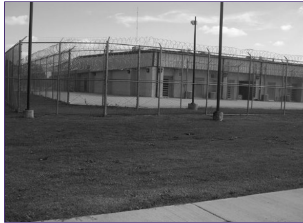
Jail with dual fenced perimeter with razor wire. (Photograph courtesy of Jim Rowenhorst.)
