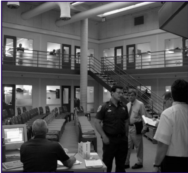
Cell fronts with large windows. Note that the bottom half of the windows are frosted for privacy in the cell. (Photograph courtesy of Voorhis Robertson Justice Services.)
